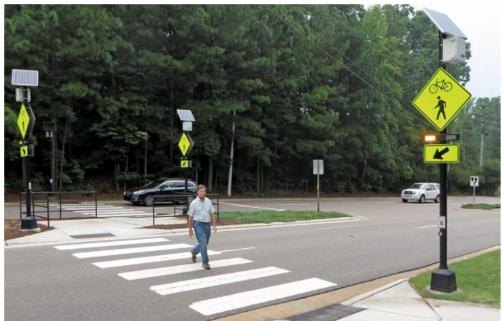
Rapid flashing beacons are motion or button activated to improve crossing visibility.
