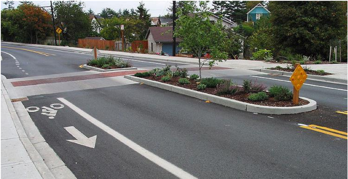
This mid-block crossing includes a raised crosswalk, colored pavement, landscaped refuge islands, and signage.
