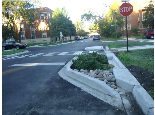
This retrofitted curb extension in Minneapolis features a supplemental storm water facility.
