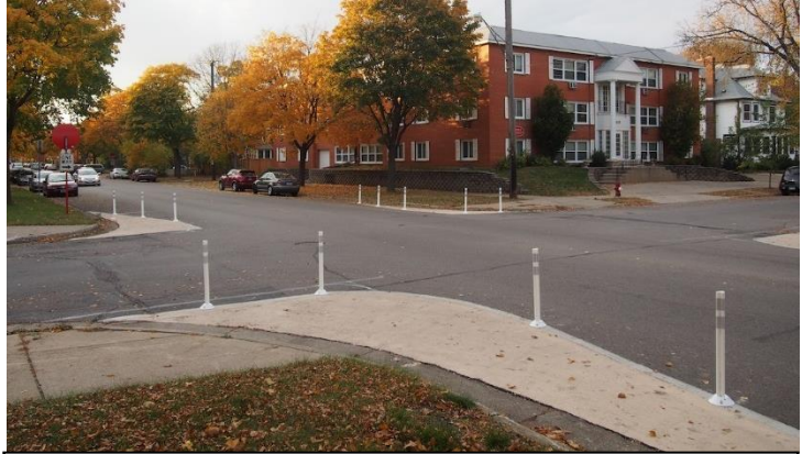
This curb extension in Minneapolis utilizes colored paint and candlestick posts as an inexpensive retrofit.
