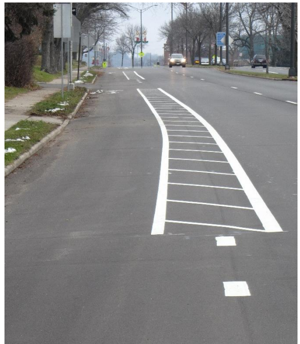
This buffered bicycle lane in Wausau, WI creates separation, with dashed lane markings through intersections.
