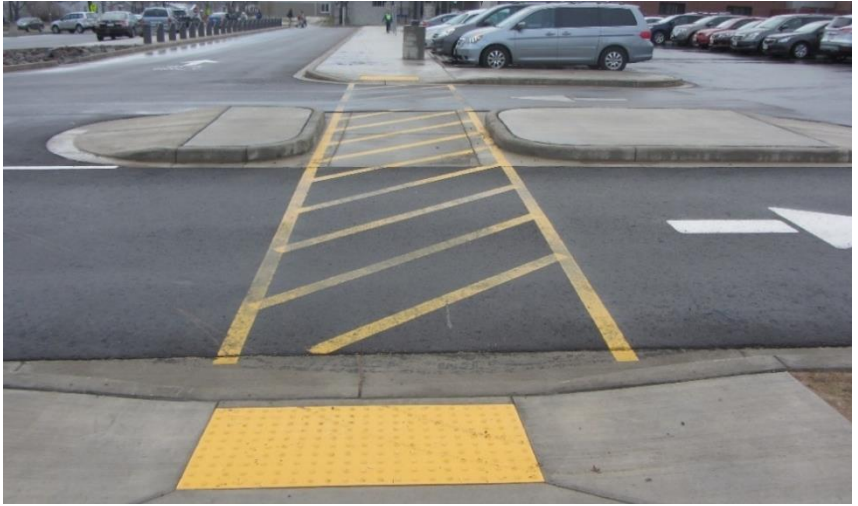
This on-site crossing of a parking lot entry of the Altoona School District Campus utilizes a refuge island and patterned crosswalk.
