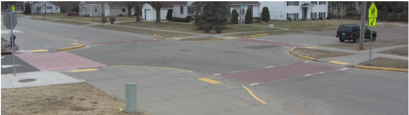
Curb extensions and colored, textured crosswalks at the Altoona School Campus improve safety and visibility in a high conflict area. This treatment was installed following recommendation of the 2009 Safe Routes to School Plan.
