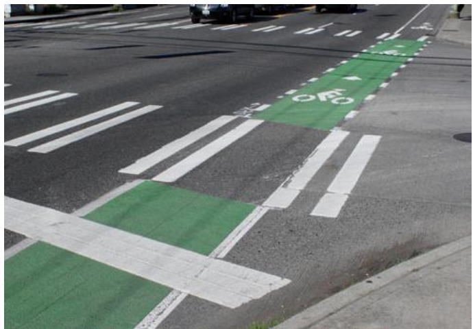
This colored and dashed bicycle lane identifies the lane of travel for cyclists through an intersection.
